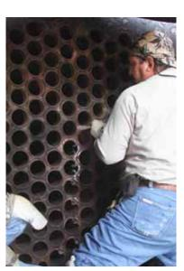
Cutting old flues loose at flue sheet.
