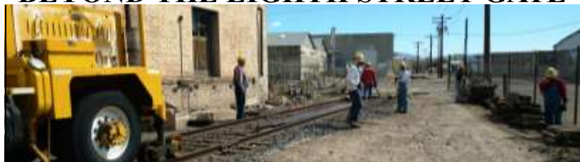
Looking East Through The Eighth Street Gate: NMSLRHS volunteers remove scrap material and clean the site at the 8th street entrance in preparation for construction of the engine house described on page 3.
