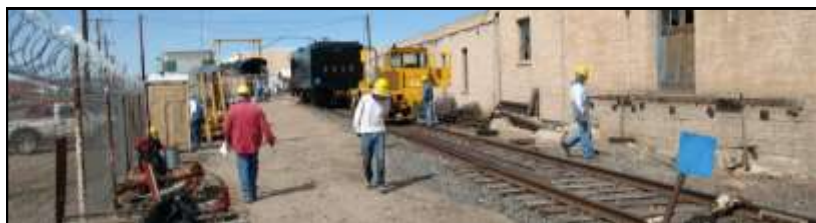
Looking West From The Eighth Street Gate: Site of the soon to be built engine house. BIA building is on right.. The GSA warehouse is visible beyond the tender and locomotive at center of the picture.
