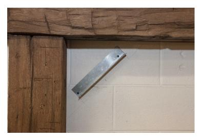
• **Step 6.** Place the knee brace over the bracket and check placement making sure mounting bracket is not holding knee brace off mantle and leg you want the 1/8" from step 4 so it will tighten up the knee brace.
