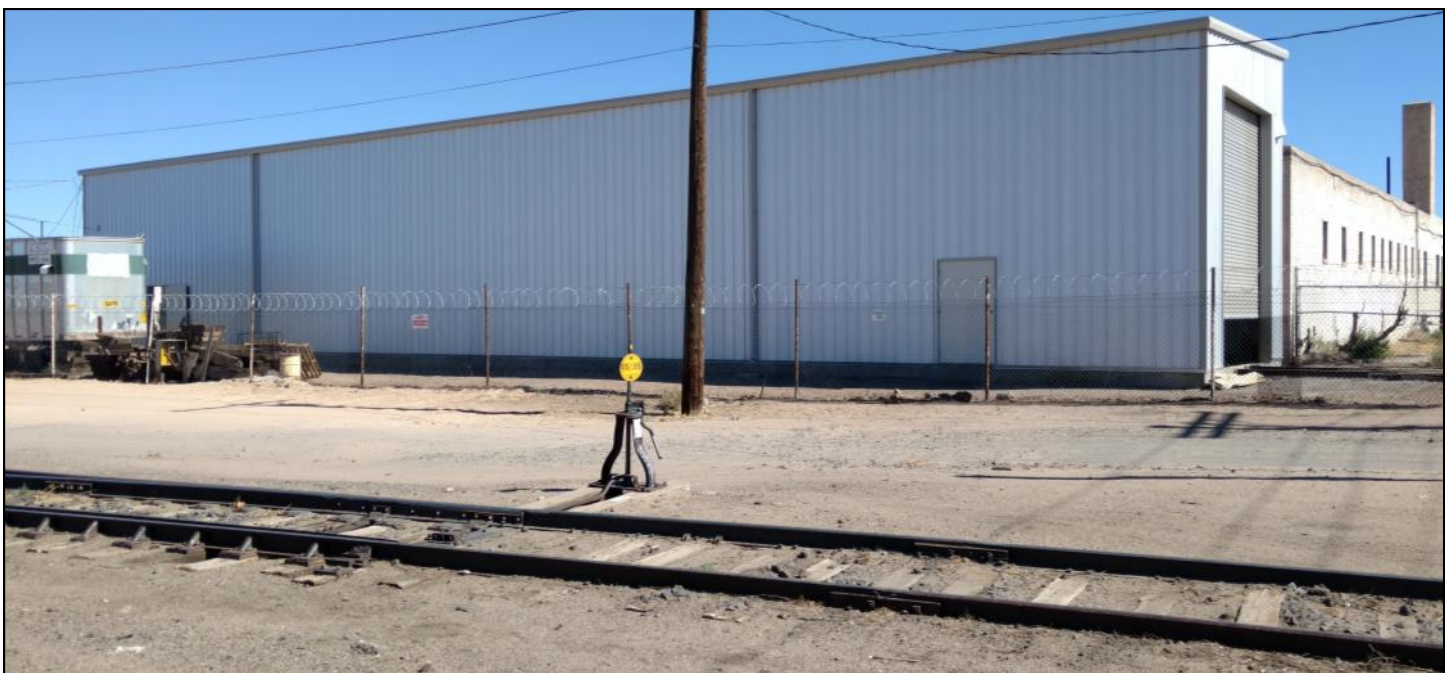
Santa Fe 2926 Engine Shed: This picture shows the new engine shed as appears to anyone traveling north on 8 th St NW at the crossing of the Sawmill Rail Spur. The building at extreme right is a BIA warehouse.
