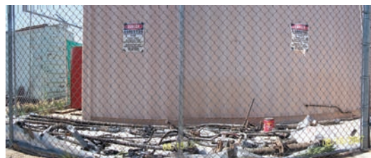
Asbestos impound area: All pipes, fittings or other appurtenances with asbestos that are removed from the locomotive are stored in this impound area awaiting GranCor remediation activity.
