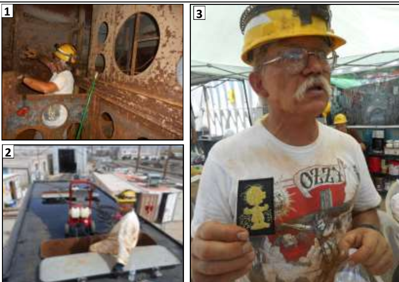
Bunker Cleaning And Preparation, Stage 1, 2003: The cleaning began in early 2003 by removing caked oil inside and out, (1 & 2). The fuel bunker was then lifted, (3) from the tender and placed on cribbing for more cleaning, Surprise!! More caked oil and assorted trash in the fuel bunker pocket, (4). Inside the water bunker, the crew scraped, scrubbed, and needle scaled hundred of pounds of scale, rust, and trash.
