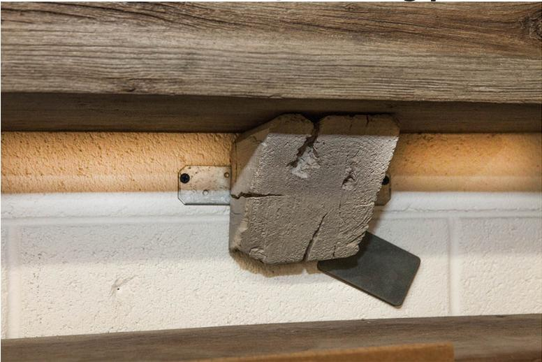
**Picture of drilled hole in corbel**
