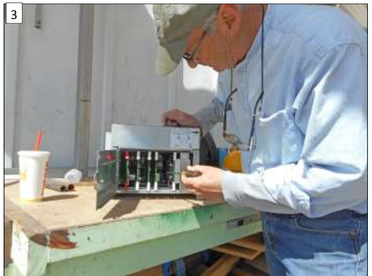
Small Box, Big Job: The small box with a handful of circuit boards is a primary control component of the 26L system.
