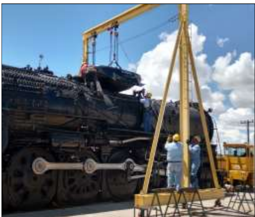
Sand Dome Installation: 'Big Bird' lifts the sand dome and eases it into place atop 2926.
