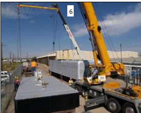
Really Heavy Lifting, Sept. 2007: Two large cranes were required to reassemble the 2926 tender—lifting the trucks onto the track, lifting the tender body onto the trucks, and then lifting the fuel bunker and dropping it into place on the tender body.
