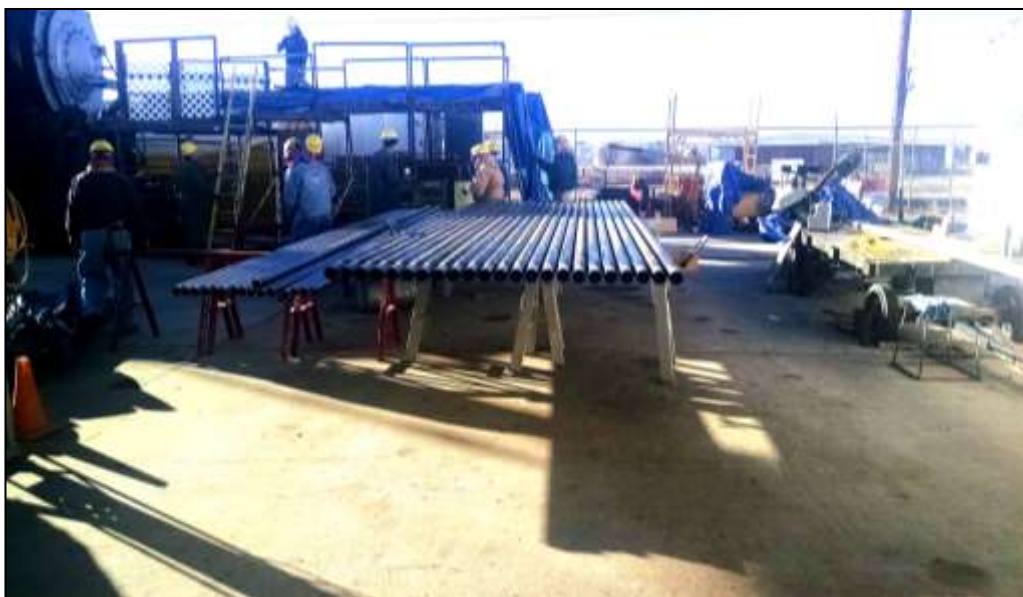
Setting Up For Flue Tube Insertion: In this picture, scaffold assembly is underway next to a rack of the first flue tubes sized and cleaned. At right is the heavy metal wagon that was pressed into use as a work table with the metal saw fastened to the end, to create a jig for sizing and trimming tubes.
