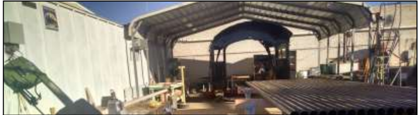
Under a canopy in the corner of the restoration site, the cab crew working on the cab's electrical has at least a bit of protection from the weather.
