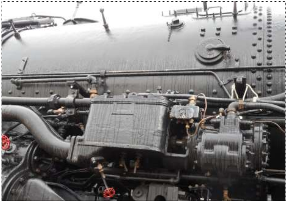
With rainwater dripping down its side, 2926 appears to be alone. The following pictures tell a different story. The 2926 volunteers do not let a little inclement weather slow their continuing work to bring the big locomotive back to life.
