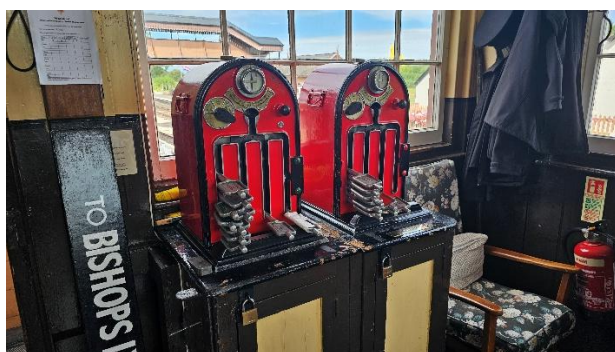
The token system used to ensure that there is only one engine on the single-line track at any time.
