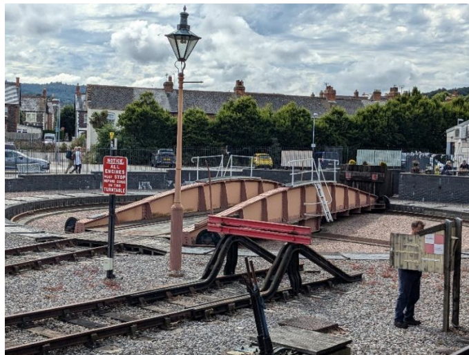
WSR's (relatively small) manually operated turntable at Minehead.
