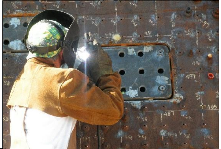
Above: Welding patches on the engineer's side wrapper sheet. Here, John G. and Danny R work (Left) inside and (Right) outside the firebox. Below: Next, on to the big patch on the fireman's side of the wrapper sheet.
