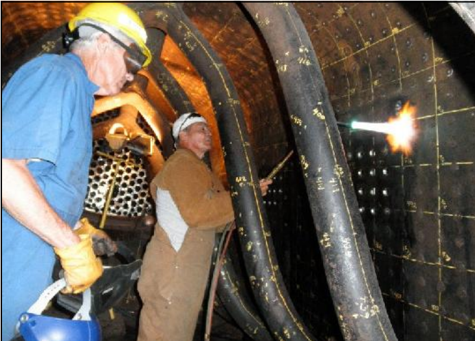
Above: Welding patches on the engineer's side wrapper sheet. Here, John G. and Danny R work (Left) inside and (Right) outside the firebox. Below: Next, on to the big patch on the fireman's side of the wrapper sheet.
