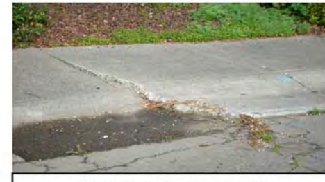
EXAMPLE: Asphalt repairs
