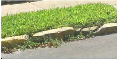
EXAMPLE: Settlement / Vertical Offset
