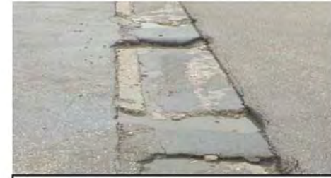
EXAMPLE: Large Holes in Surface
