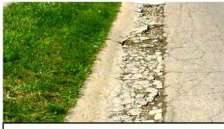
EXAMPLE: Exposed aggregate
