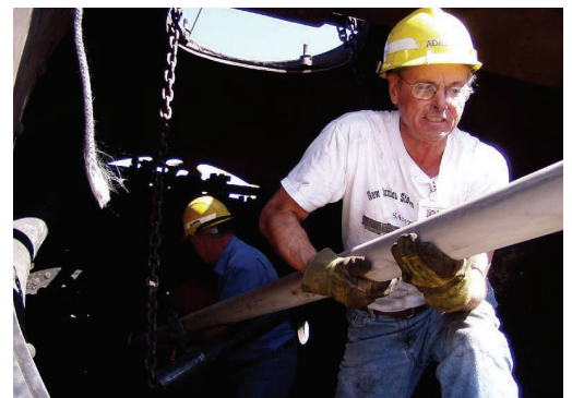
Working in the 2926 smokebox, Pete helps pull one of the huge locomotive’s flue tubes.
