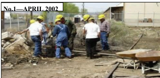
Cleaning GSA/BIA Lots & Siding For 2926's New Home
