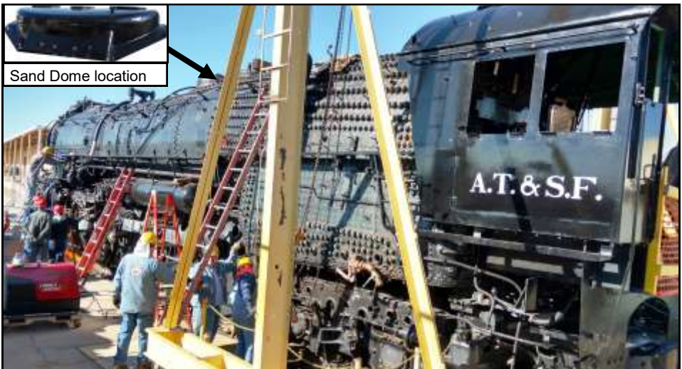
Busy crew at work reinstalling appliances: The finished sand dome is shown in the inset. At 10 feet long, 6 feet wide, and weighing almost half a ton, it will be lifted by the gantry crane and installed just behind the steam dome, (arrow). A stepladder and another small ladder are next to an air tank that has already been installed.
