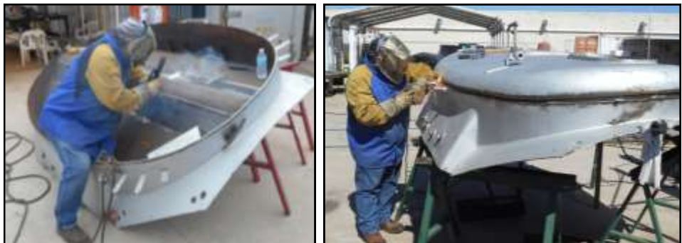
Master welder Carlos Osuna works on a total rebuild of the 2926 sand dome.
