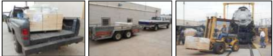
Late October, 7511 pounds of refractory material (firebrick) arrives on site.
