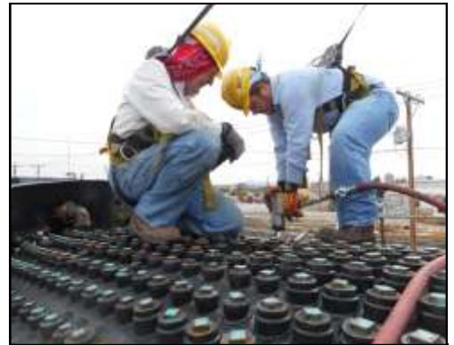
Finding and Fixing Those Pesky Leaks: 1. With 125 lb air pressure on the boiler system, Dave and Bob spray soapy water on neatly installed stay bolts. 2. Some leaks can be sealed with just a bit more torque on the bolt.
