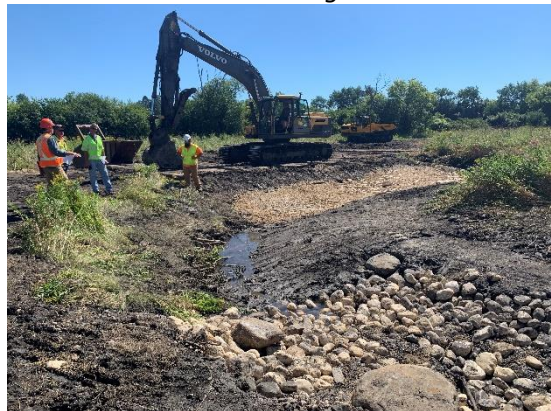
Site Photos – August 31 st
