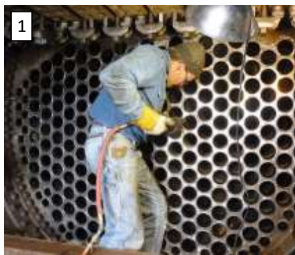
Welch boiler specialists at work: Photo 1, rolling tubes on the front flue sheet. The U-shaped devices at top are Superheater clamps. Photo 2, rolling tubes on the rear flue sheet. Ernie RobartPhotos:
