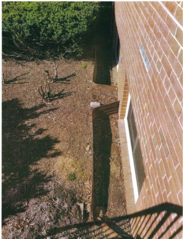
Old window wells
