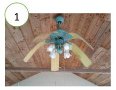
Ceiling Fans – make sure they are operating and remotes have new batteries. If the blades "droop" the fan will need to be replaced.
