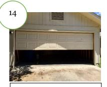
Test the garage door to be sure the auto reverse is functioning properly.
