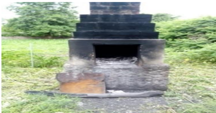
Defective incinerator used for health care waste disposal.
