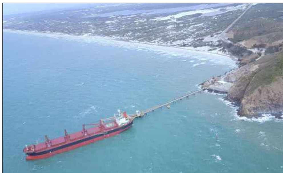
Figure 6: Ports North jetty and Mitsubishi ship-loader
