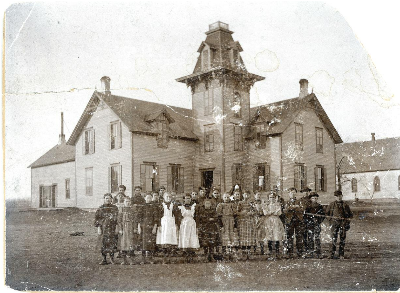
The parochial school, St. Joseph Catholic School, was built in 1885, near St. Joseph. Pictured are students standing in front of the St. Joseph Catholic School. This photo was taken before the fire that destroyed the original frame church in 1908 (visible on the right side of the photo). Register archive photo
