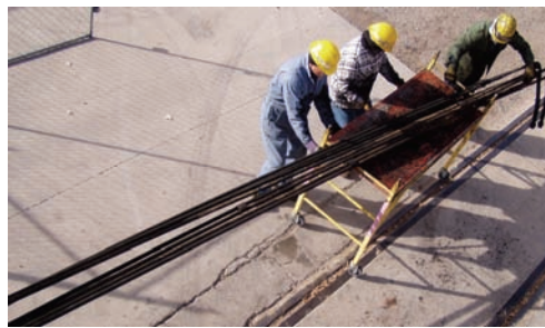
Another bundle of super heater pipes heads across the concrete to a storage rack.
