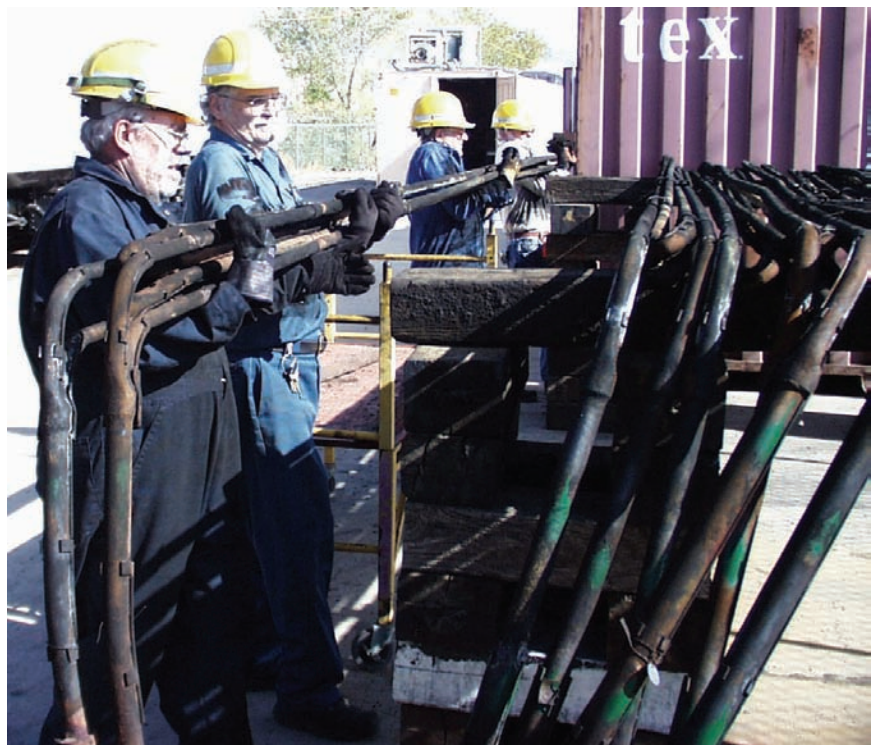
Steve Bradford, Lawrence Harmon and Dave Traudt lift a pipe bundle onto cribbing.
