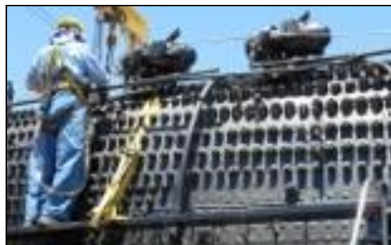
Almost There: The piece of pipe being painted has been bent to fit the place it will be installed, fittings have been added. With such a crooked pipe, the final step, installation, may require a bit of manipulation.
