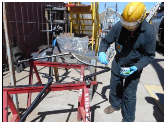
Almost There: The piece of pipe being painted has been bent to fit the place it will be installed, fittings have been added. With such a crooked pipe, the final step, installation, may require a bit of manipulation.
