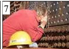
**To Be Continued:** Soon, welder Danny Rivera will begin the delicate process of welding the patch into place. The resulting patch must be strong enough to withstand the boiler pressure of more than 300 psi.
