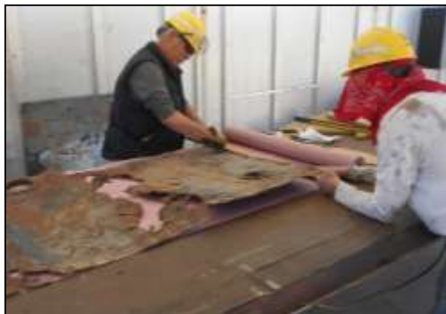
Right & Above: Sheet metal jacketing parts pulled from storage. The numbering helped, but the pattern making crew was still faced with a challenge.
