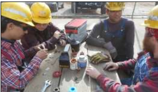
Left to Right: Scotty, Teddy, Anthony, and Henry chat while working on small valve parts. These young agile volunteers are more often seen atop or underneath 2926 in hard to reach spaces.
