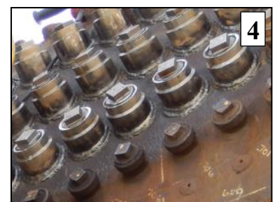
Repair and Replacement parts: (1) A selection of new staybolts. (2) New staybolt cap parts. Lower picture shows installation of copper gasket that was used in staybolt cap assembly. (3) Flexible staybolt assembly (4) Completed staybolts alongside original flexible and fixed staybolts.
