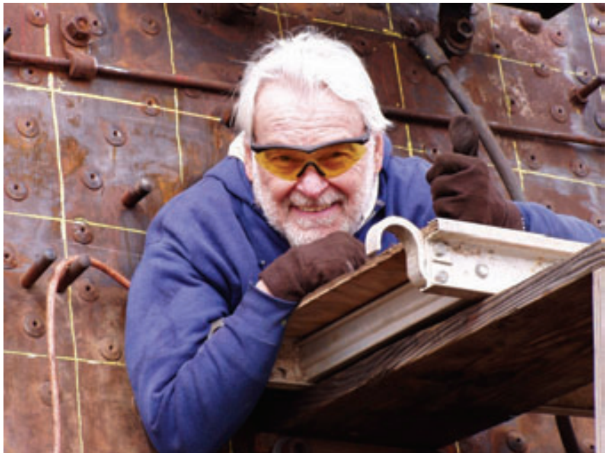
Randy McEntire emerges from the firebox where he has been drawing grid lines to be used in the UT process. Ultrasound readings will be taken at the line intersections. The readings will be used to determine points at which boiler repair may be necessary.
