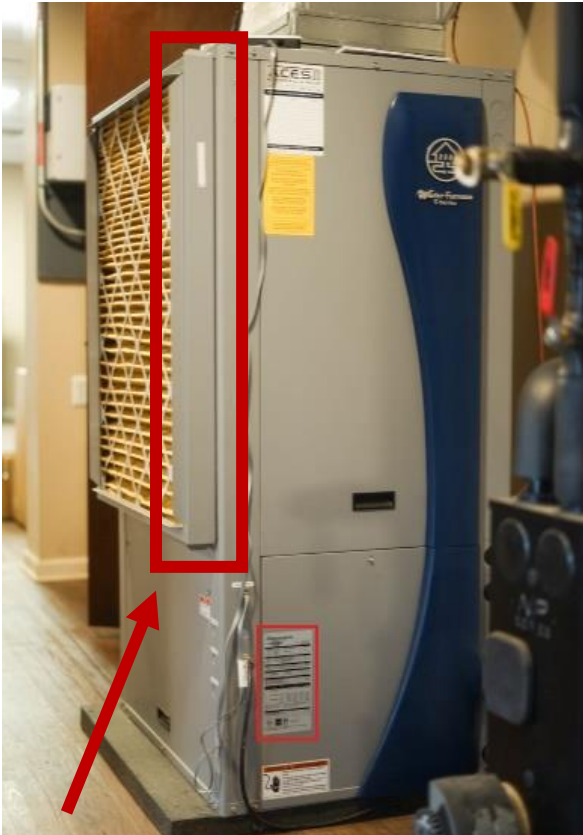
Remove filter housing door
