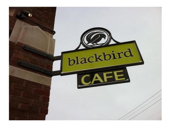
Machine cut sheet metal over framed, painted metal
