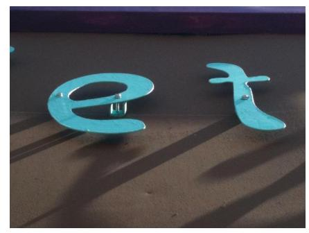
Machine-cut metal; off-set mounted
