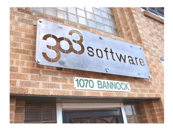
Machine cut sheet metal; offset from facade
