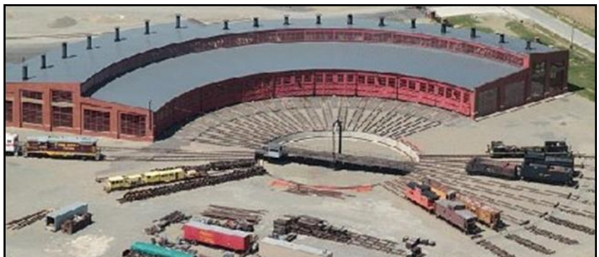
Typical turntable and roundhouse layout: The turntable at the AT&SF Rail Shops in Albuquerque is functional. The roundhouse will be rebuilt. Check our web site http://www.nmslrhs.org to view proposed floor plan, elevation, and further information on our plans for the future home of 2926, and the coaches it will pull for excursions—excursions that will allow New Mexicans and tourists from everywhere to experience a bit of our state's rich railroad history.
