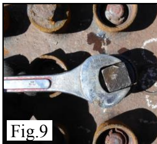
ALL staybolt assemblies must be cleaned, inspected and have a new copper sealing washer installed. Those components that are deteriorated beyond reuse must be replaced. Parts that are to be reused are cleaned and held for reassembly.
