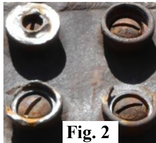
Staybolt assemblies vary. Parts of some staybolt assemblies and deterioration examples are shown above. Fig. 1 shows three types. The first (A) shows a three piece assembly with the bolt head seated in a removable sleeve with a threaded cap. In a two piece type, (B) the seat is permanently fixed on the boiler wall. Two types of crown sheet staybolts are shown in (C). In Fig. 2, at least three (and maybe all four) of these staybolt assemblies will require some parts replacement. Variations go beyond just length or fixed versus flexible. There are also different sizes of sleeves and caps. Fig. 3 shows some of the replacement parts.
