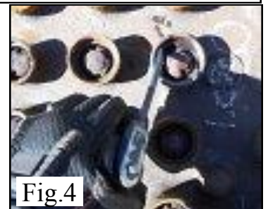
ALL staybolt assemblies must be cleaned, inspected and have a new copper sealing washer installed. Those components that are deteriorated beyond reuse must be replaced. Parts that are to be reused are cleaned and held for reassembly.
